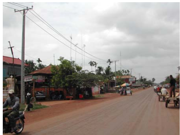
Medium Voltage System after Improvement
